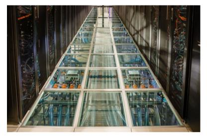
Sandia National Labs deployed two supercomputers equipped with Chilldyne's negative pressure liquid cooling system, operational since 2019 with zero leaks.
