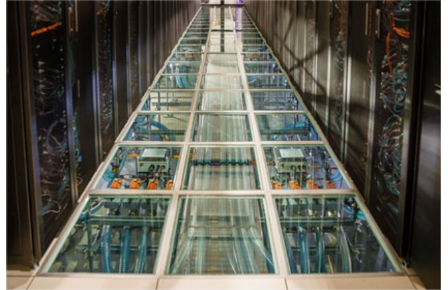
The supercomputer at Sandia National Laboratories with the under-floor automatic switchover valves that enable the system's N+1 smart redundancy to maximize uptime.
