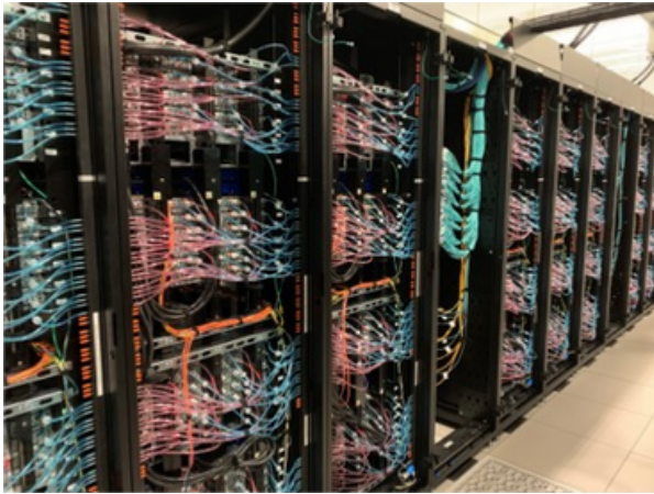
OCP Rack Manifold at Sandia National Labs
